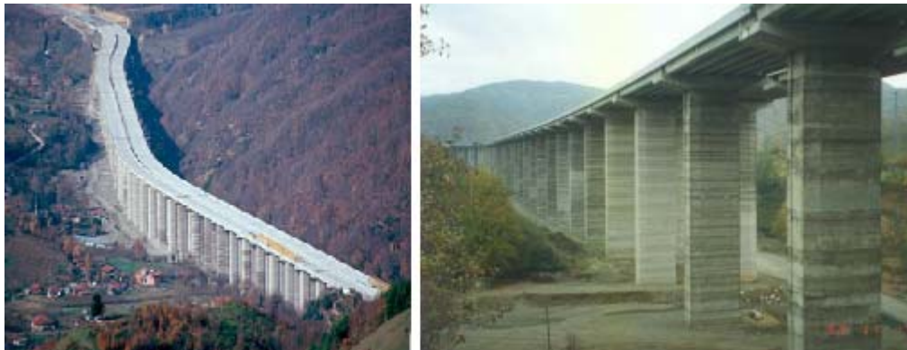
Figure 3: General view from the Viaduct 1
